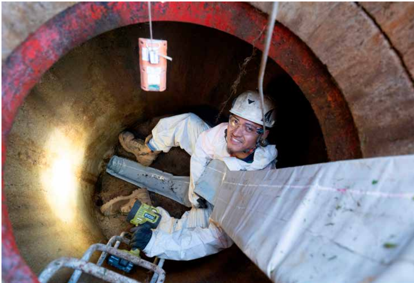
Relining the Coast's underground pipes involves inserting a flexible liner into a pipe via one manhole, which is then pulled through to the pipe's next manhole. Image / Watercare.
