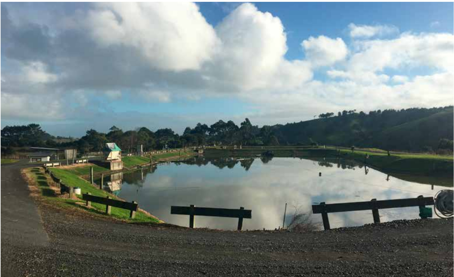
A digester pond at the Beachlands Wastewater Treatment Plant. Image / supplied.
