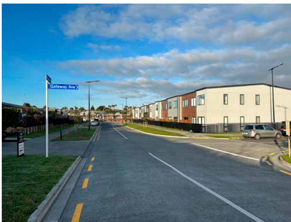
The new road connecting Beachlands to Pine Harbour (Winterman Way, pictured above) has opened, but ferry commuters will have to wait until 2025 for a bus service connecting the two areas.
