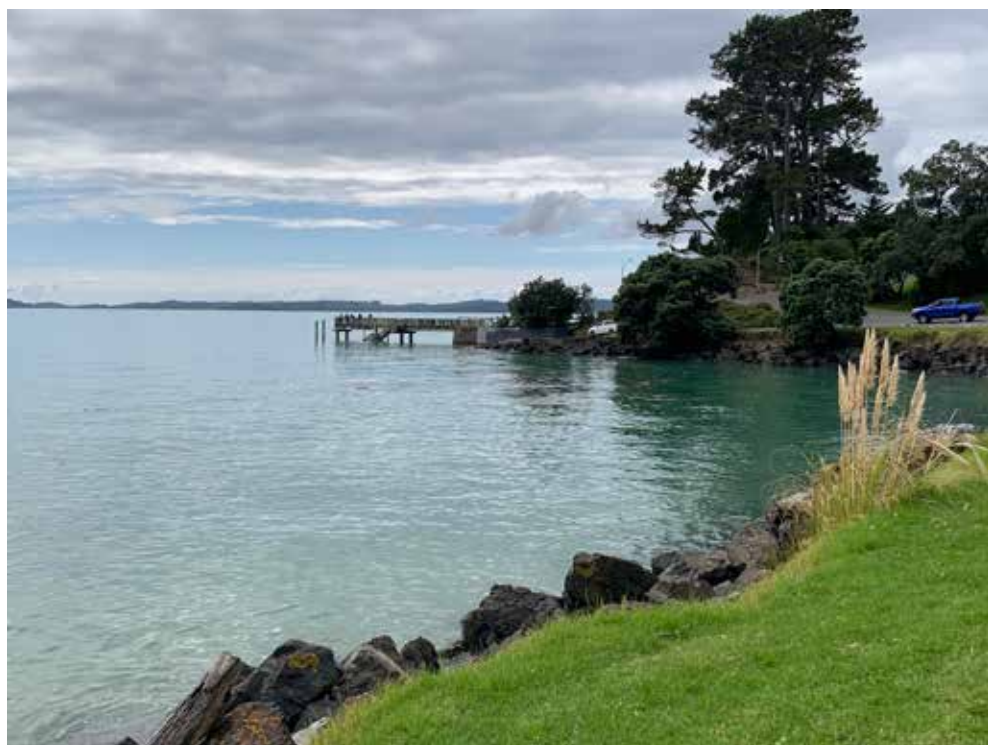
Work will start next year on replacing the eastern end of Sunkist Bay's seawall.
